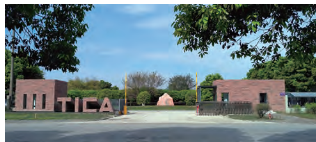
Chengdu factory Construction area of 20,000 square meters
